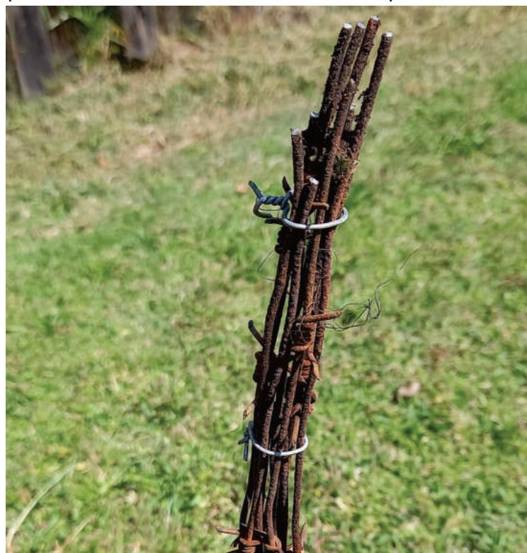
Close-up of a dropper made from scrap barbed wire, showing bindings to hold the rusty strands tightly together.
