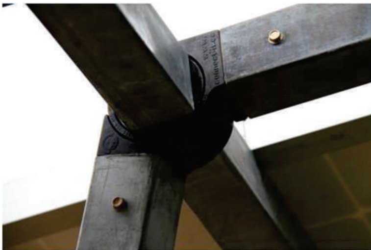
Adjustable fittings enable any angle to be constructed.
