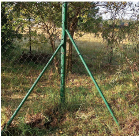
Steel corner post (centre) with a stay on either side to form a right angle.
